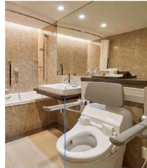
Outlet underside of the basin
