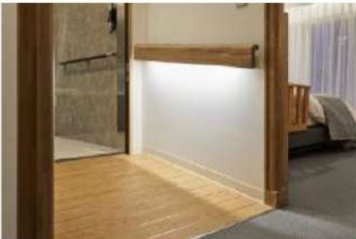
Slope to the bathroom
